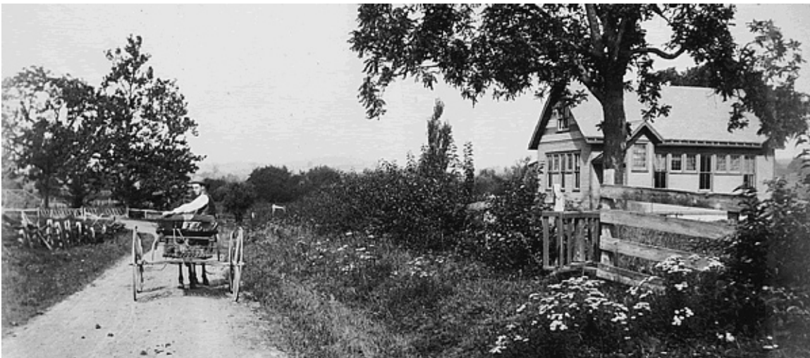
This photo of the Pleasant Valley Schoolhouse shows the east wall windows consisting of three vertical windows with upper windows in between making almost a complete wall of windows. This is quite different from the usual simple three vertical windows. In the 1874 plan there were only two vertical windows.
