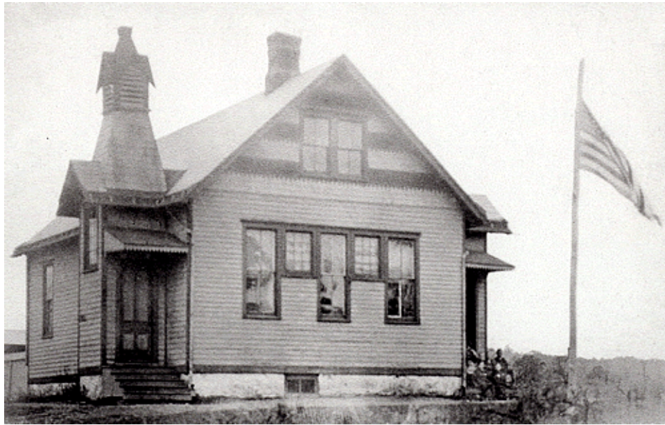
This photo of Pleasant Valley 1889 schoolhouse shows the modifications such as moving the bell tower, modifying the window plan, and much less decorative trim.
